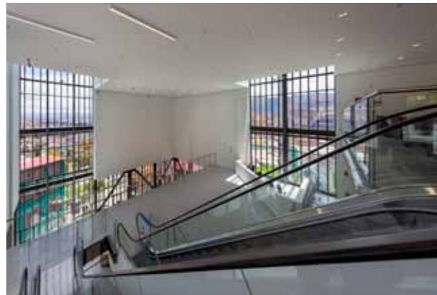
pic_05: The grid of the external sun protection determined the size of the glass elements, which are usually 1.20 m x 2.40 m. pic_07: The versatile modular system from Jansen VISS also enabled the seamless transition from the façade to the roof glazing.
