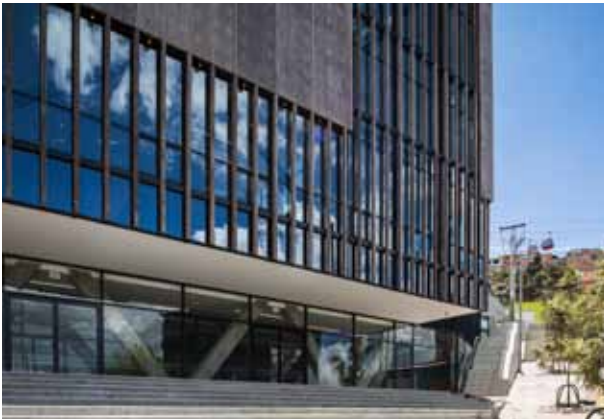
pic_04: Ground floor: Façade in Economy 50 steel system (doors and fixed glazing); doors with panic evacuation systems. Above: VISS Basic curtain wall (with inlaid windows of Economy 50). The steel structure supports the sunshade system made from concrete slats.
