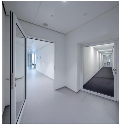
pic 03: The T30 fire doors in the rental areas are generally 226 centimetres high.
