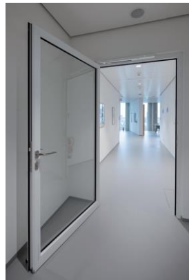
pic 06: ... continue the light impression of the façade inside.
