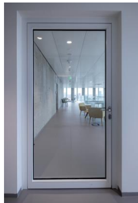
pic 05: White powder-coated tubular steel frame doors
