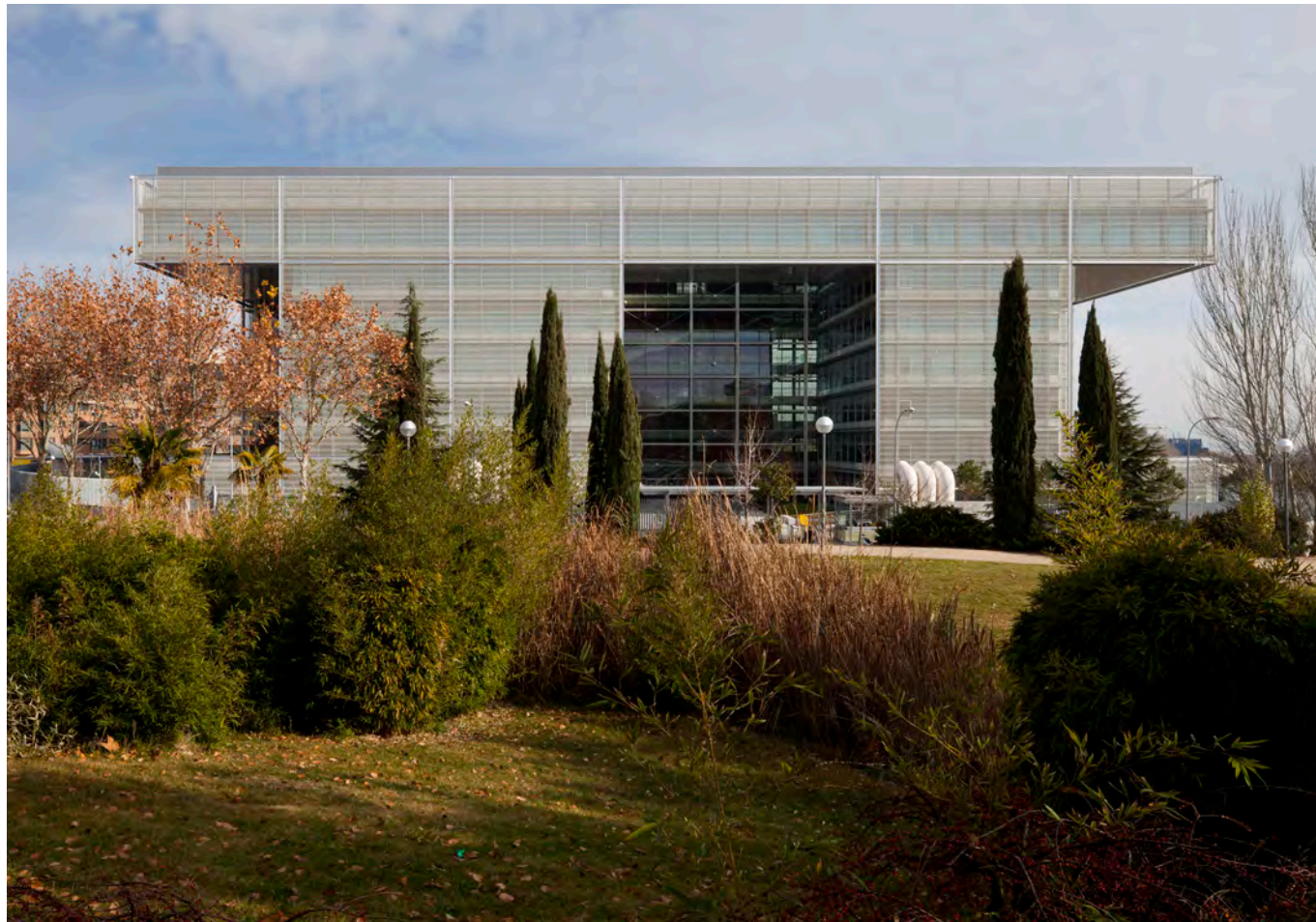
The ceramic coating on the solar reflector tubes in front of the outer façades catches the light and diffuses it into the building at a dimmed level.
