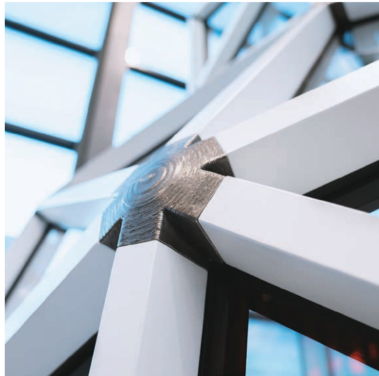
VISS 3 3D printed steel nodes
