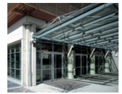
Montage Montage Installation
